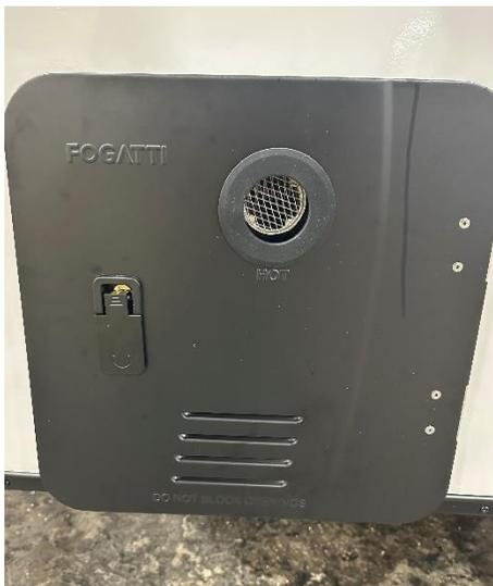
The most common trouble with electric water heaters results from energizing the water heater before it is filled with water. Even brief operation of the electric element without water in the tank will burn out the electric heating element.
