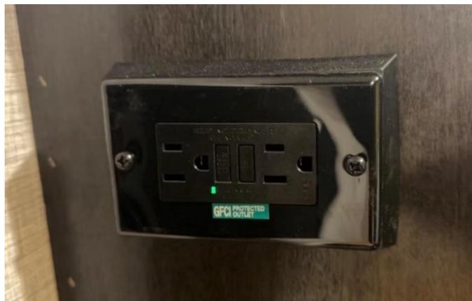
This GFCI receptacle will not protect against short-circuits or overloads. The circuit breaker or fuse in the electrical panel which supplies power to the circuit provides this protection.
